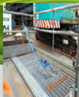
Remove grating with approved hooks &amp; secondary snaphook
