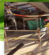
Barricading below working area ( Danger soft tape ).
