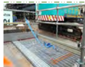
For moving of grating use Approved hooks and secondary snap hook lanyard
