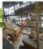
Must wear full body harness 100% tie off when working
