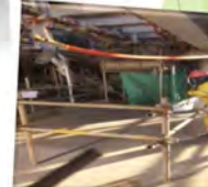
Isolating of below working area with hard or soft barricading red danger sign and standby man
