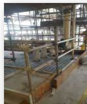
hard barricading on the working area
