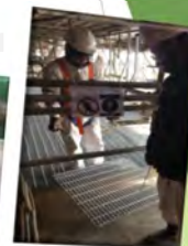
Isolating of working area with hard barricading
